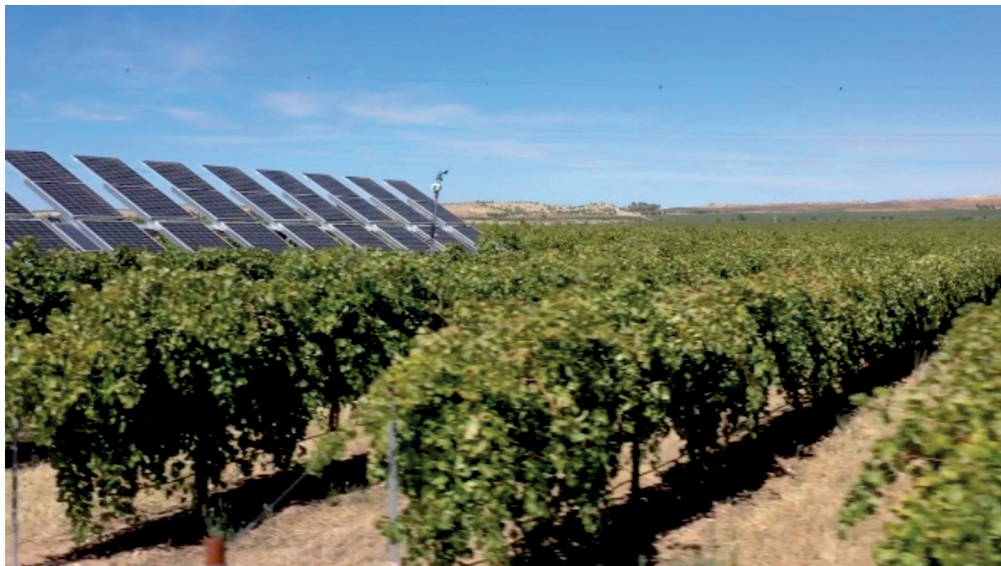
Figure 17 First smart agrivoltaic plant in Spain (Guadamur, Toledo)
