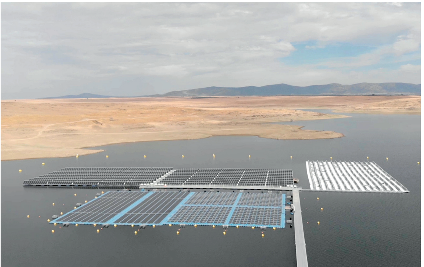
Figure 36 Sierra Brava floating photovoltaic plant
