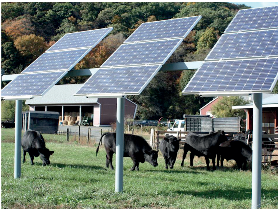
Figure 30 Cows grazing the grassland under the solar power plant
